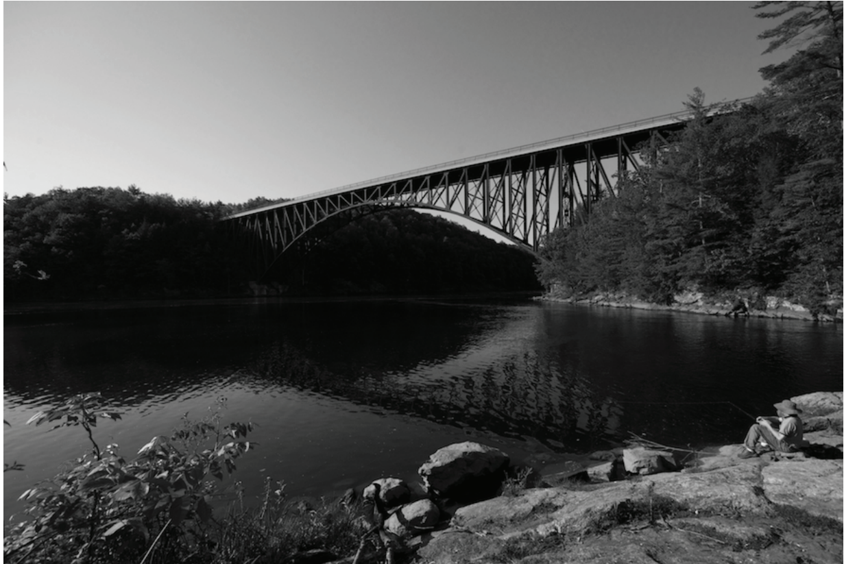
French King Bridge Over Connecticut River - Erving
